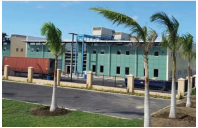
Barnett Tech Park Lot 3 in Montego Bay completed in 2015 (Method of Construction: Steel framed building with insulated panels)
