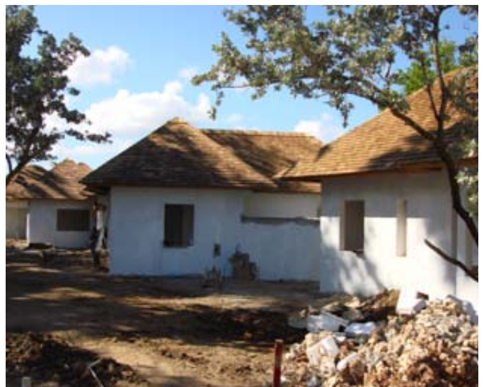
Trident Cottages Phase 1 completed in 2008 (Method of Construction: Block and steel)
